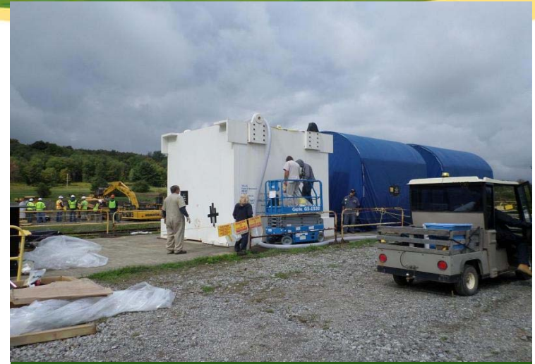
Melter Grouting Operations
