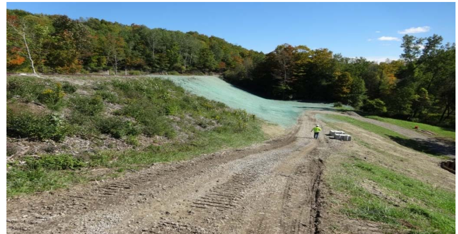
Completed Repairs to the Buttermilk Creek 90-Foot Slope
