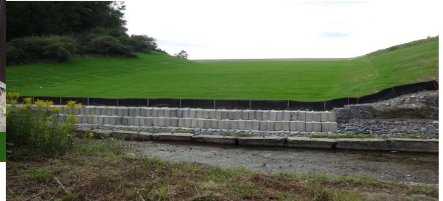
Lake 1 Spillway After Repairs
