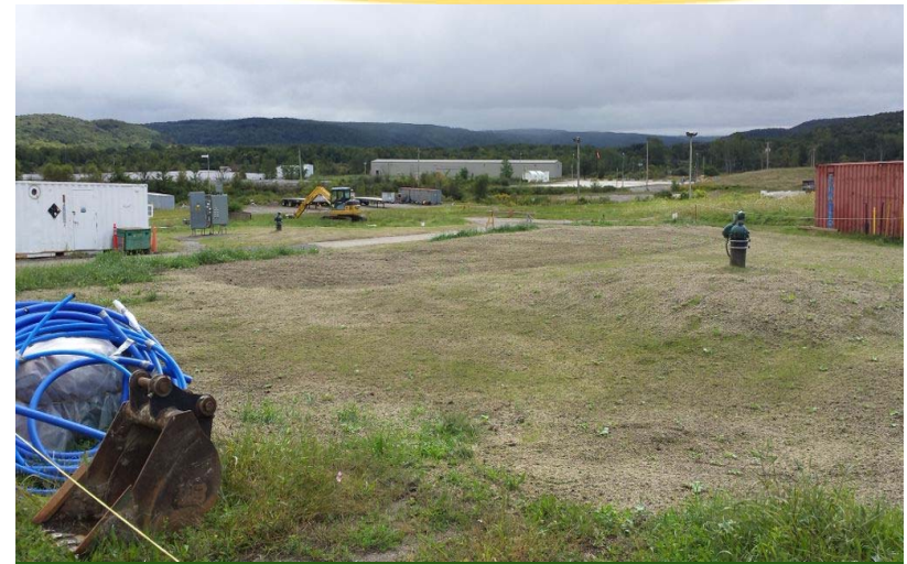
Completed Wells 1 and 2
