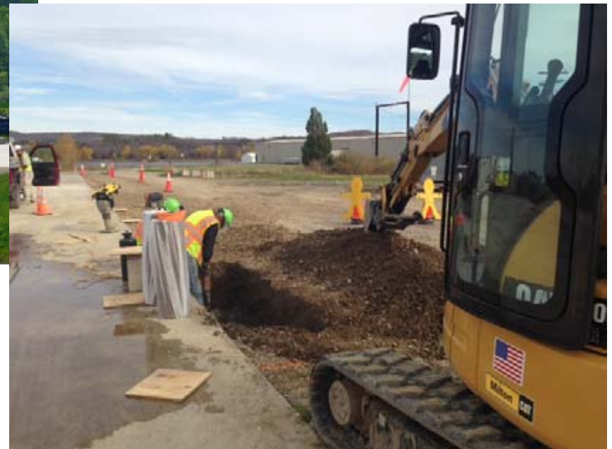
Excavation and Installation of Security Fence
