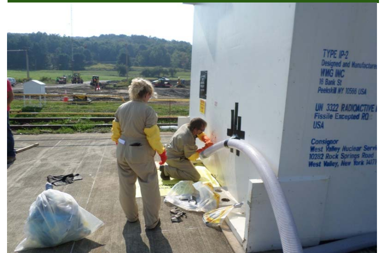
Melter Grouting Operations
