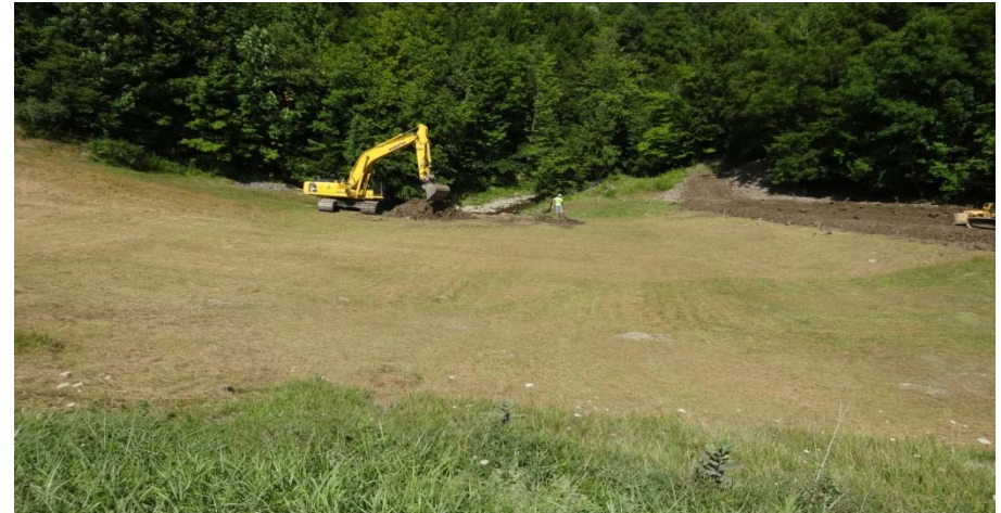
Starting Repairs at Base of Lake 2 Dam
