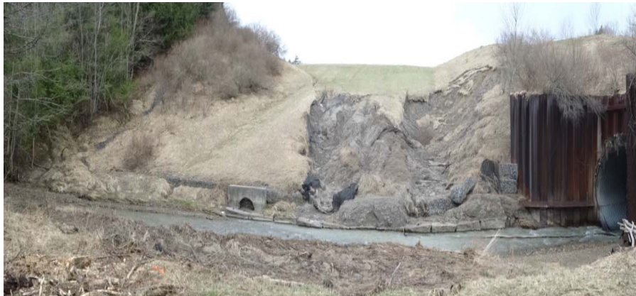
Lake 1 Spillway Erosion Before Repairs
